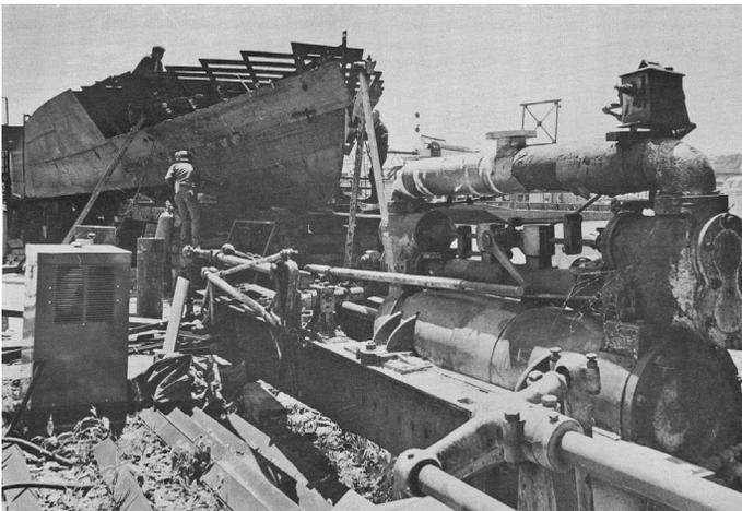
*Upper two photos show CITY OF BATON ROUGE on March 21, 1970 at Dubuque Boat and Boiler yards as work progresses on salvaging her engines and paddlewheel assembly. In bottom view, her engines wait to be placed aboard JULIA BELLE SWAIN, while hull plating nears completion in the background. CITY OF BATON ROUGE had been renovated by this time and taken to Peoria. Photos from Editor's collection.*
