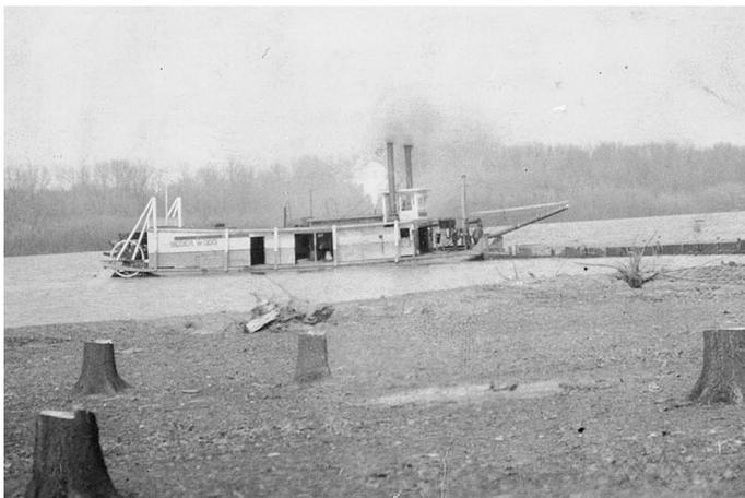
**BEDER WOOD (To216)** was another 1915 Dubuque-built boat with G&E engines 10's - 5 ft. stroke. She is pictured here doing construction work of Upper Mississippi locks and dams in the 30s. Timber on these islands was hand cut with cross cut saws before the pools were raised, leaving a forest of stumps.
