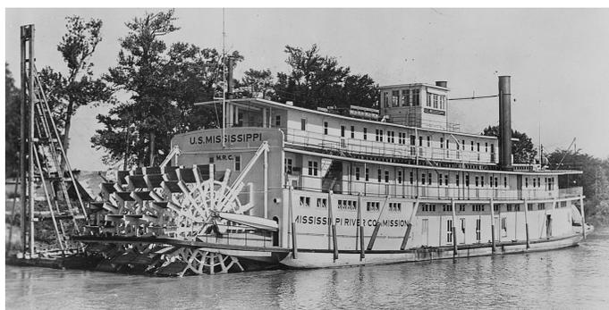
USE inspection boat **MISSISSIPPI's** engines were built by G&E in 1924 and were placed aboard at Paducah in 1927 after the hull was completed by Howards. They were 15's, 32's - 7 ft. stroke. A replacement cylinder was manufactured in 1934, the last steam engine replacement part the company ever produced.
