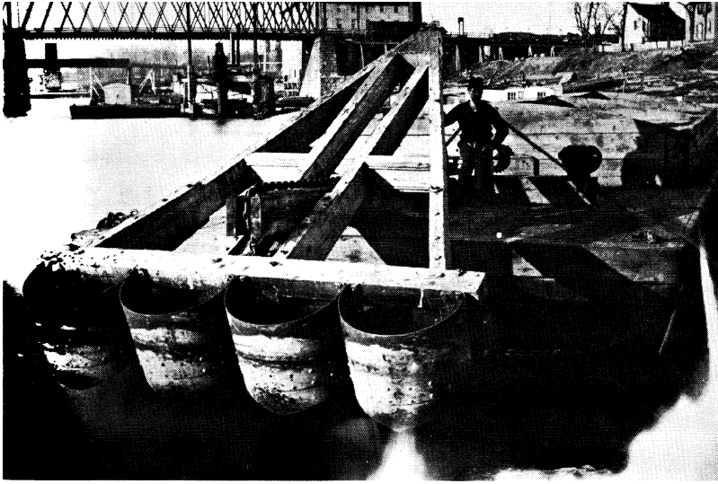
This ingenious mud scraper was designed and built for clearing mud from Muskingum River canals, locks and channels. It was handled by the VEGA and by her predecessor, an earlier VEGA built in 1881.
