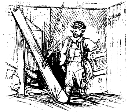
Engineer on duty; two feet of water on the lower deck.
