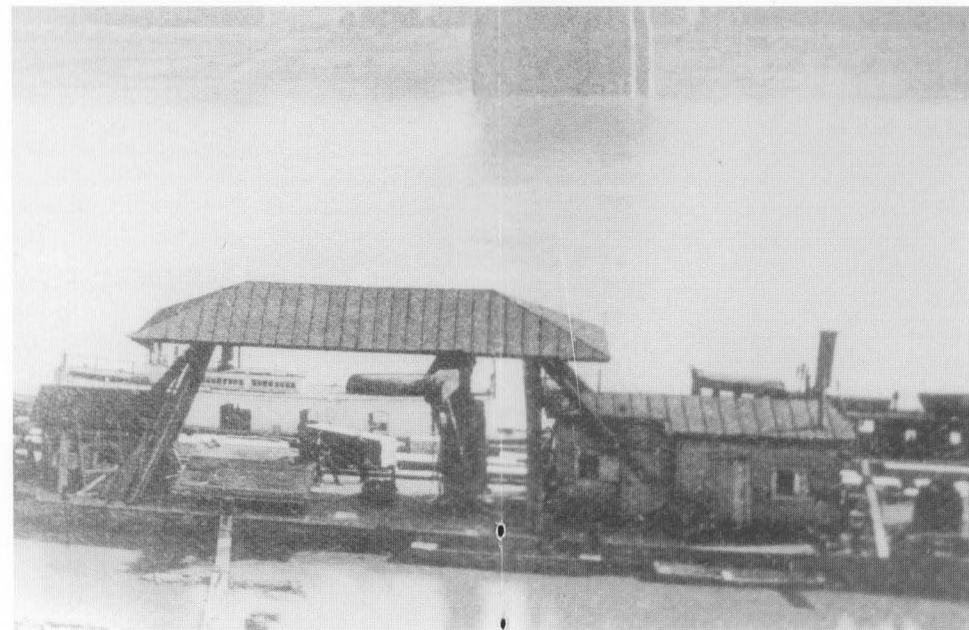
The stone boat close-up better reveals its purpose; a floating, steam sawmill for stone. A pile of sawn pieces is on the far side of the work floor, to be moved onto the flat alongside. Quarry blocks were custom cut for local buildings, street curbs, etc. and the Suspension Bridge piers.
