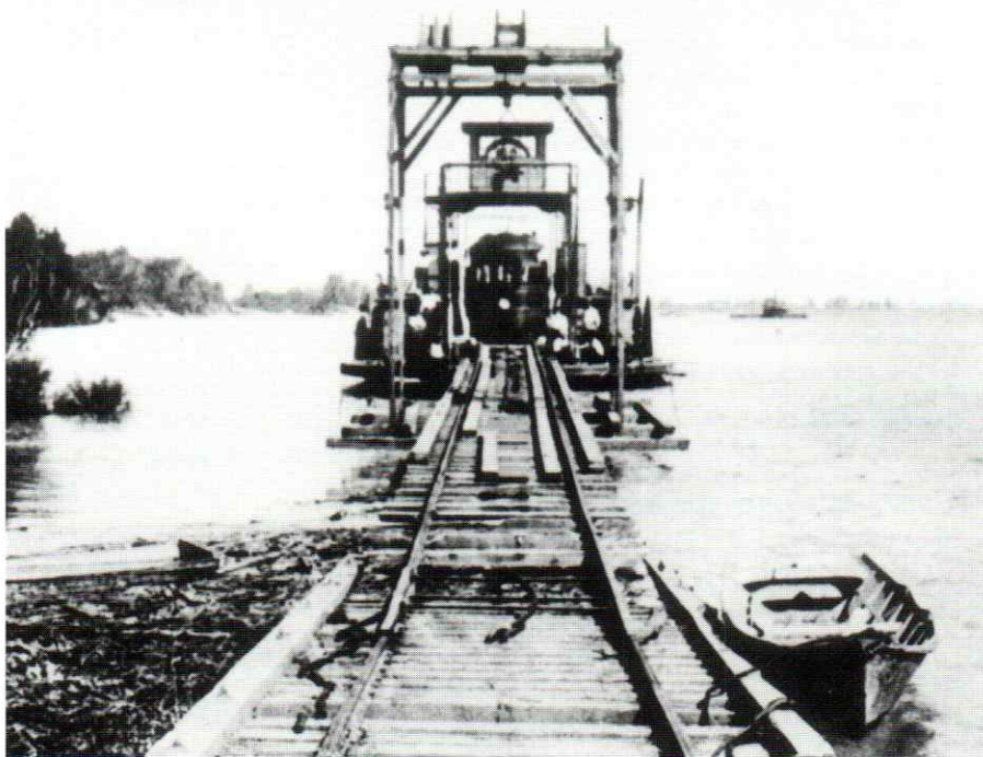
The HENDERSON at the incline on the Kentucky side of the river with an interurban car ready to come off. The ferry was single track, long enough for two cars. Photos from C. Leonard Schlamp, Evansville.
