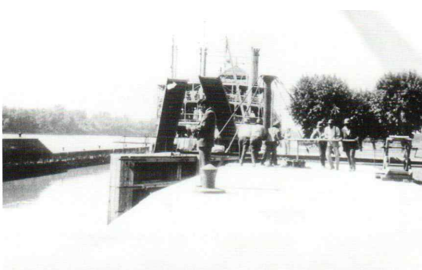
The CAPE GIRARDEAU preparing to enter an unidentified lock on the Illinois River, 1933. In the foreground is Joseph E. Vollmar, apparently studying the slow movement of the lock gate as six lockmen in background crank it open by hand.
