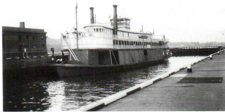
May 24, 1939, Dashields Lock. TOM GREENE on her way home after overhaul at Dravo's; new hull, new stairway, larger wheel and fresh paint.
