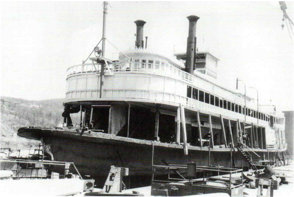
This photo of the TOM GREENE on the Dravo Marine Ways was taken on April 19, 1939, an unusually cold day with wet snow on the ground. The new hull is nearing completion; a welder is working on plates around the stem. The steel main deck was replaced by fir planking and the boiler deck strengthened for automobiles. A new outside stairway to the boiler deck and roof is yet to come. Photograph by William E. Reed.
