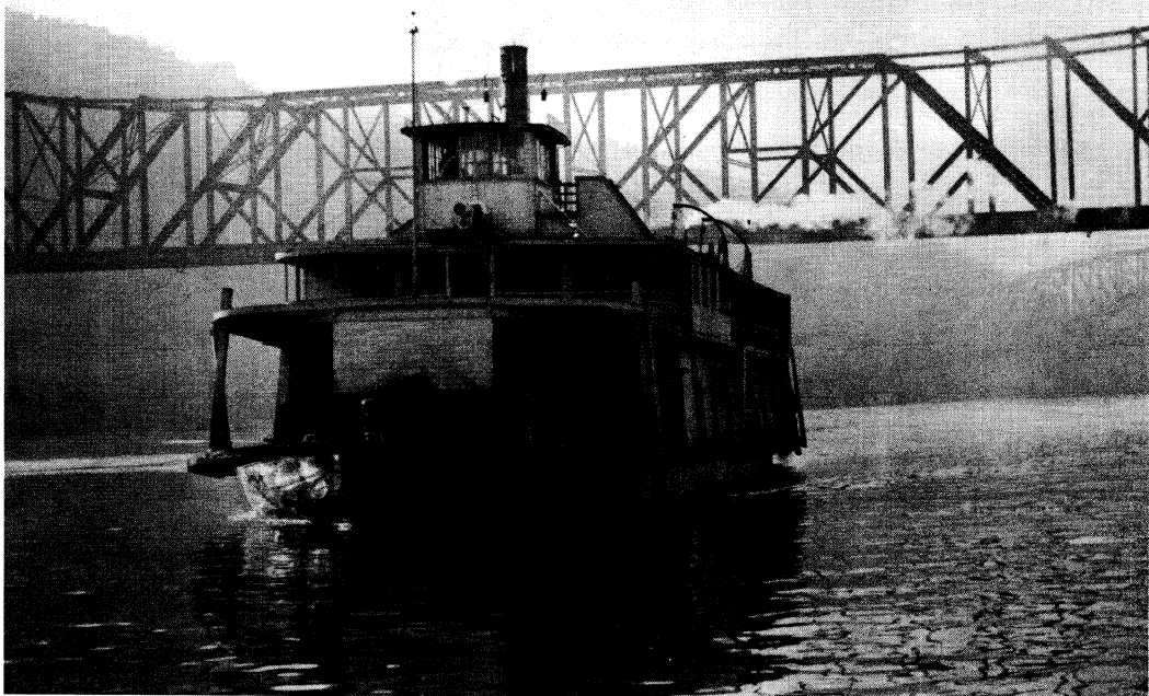
Work on the EVERGREENE was completed and trial trips run on January 14, 1936. Her only appearance at Pittsburgh was the following day when she came up to the Monongahela Wharf and picked up 86 tons of freight. The increased freeboard is evident; Wabash RR bridge behind.
