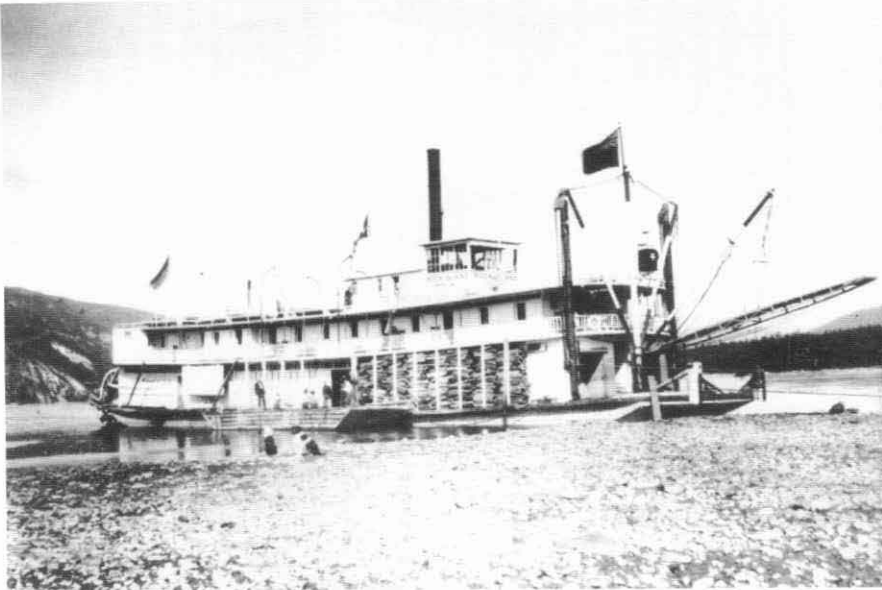
Another view of the ROCK ISLAND NO. 1 when new. Note the cargo and spar handling booms rigged on the center mast with the landing stage boom. Arthur Knutson collection.
