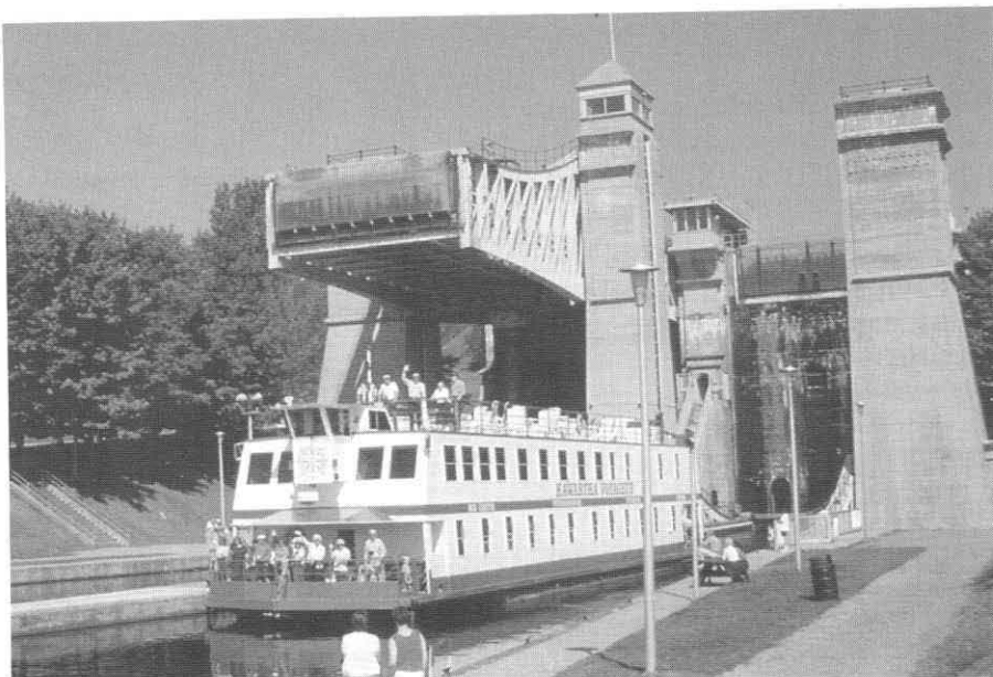
The Peterborough Lift-Lock with the KAWARTHA VOYAGEUR just exiting the lower "tub". Completed in 1904 with towers 100 ft. high of monolithic concrete, the lift is 65 ft. The pilothouse of the boat projects from the second deck lounge. Style is, "Form follows function."
