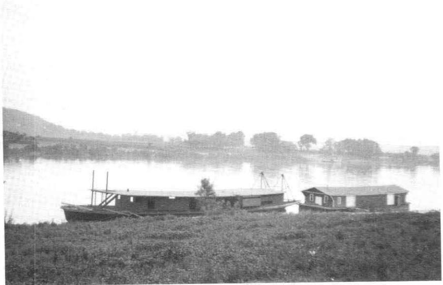
Early in June, 1924 the completed hull of the "New Boat" was towed from the Ward yard at Charleston to the Acme Boiler landing below Gallipolis. The steel work completed by Wards included the main and boiler decks. C. C. Bowyer photo.
