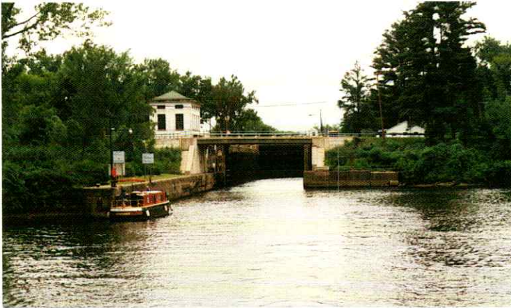
Lock 5, Champlain Canal (Hudson River) from the downstream side; lift 19 ft., dam off right.
