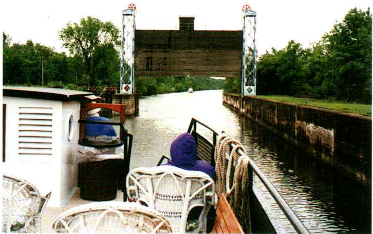
No, not a guillotine; a guard gate to protect canal when the river stage is high. Entrance to canal leading to Lock 6, Champlain Canal.
