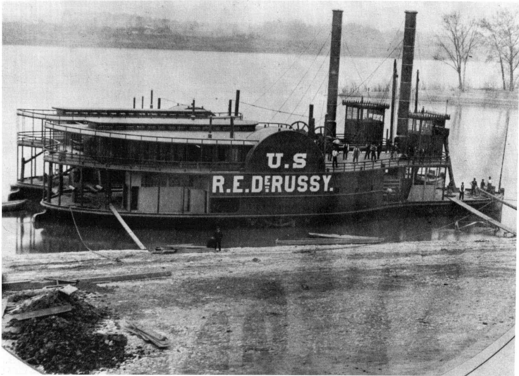
R. E. DeRUSSY (T2088A) just completed at the Portland, Kentucky landing, April, 1868. She is built almost as two separate boats, twin hulls, twin pilot houses, twin rudders, etc. The rollers for carrying
