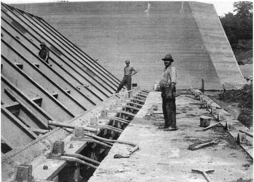
The diary mentions a number of locks and dams under construction during 1915. Here is the scene at Dam 29, Ashland, Kentucky on August 27 showing a bear trap completed and in the "down" position.
