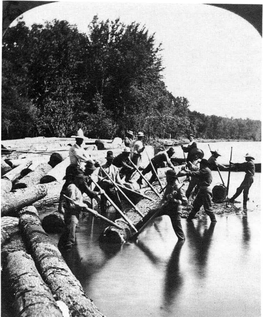
A group of log drivers on the St. Croix River pause while J. P. Doremus takes an "instantaneous" picture. Logs have piled up on a sandbar, possibly below St. Croix Falls, and the peaveys are being used to roll them back into the stream. The "peavey hook" was named for Joseph Peavey, its inventor. From the Mary Green collection.
