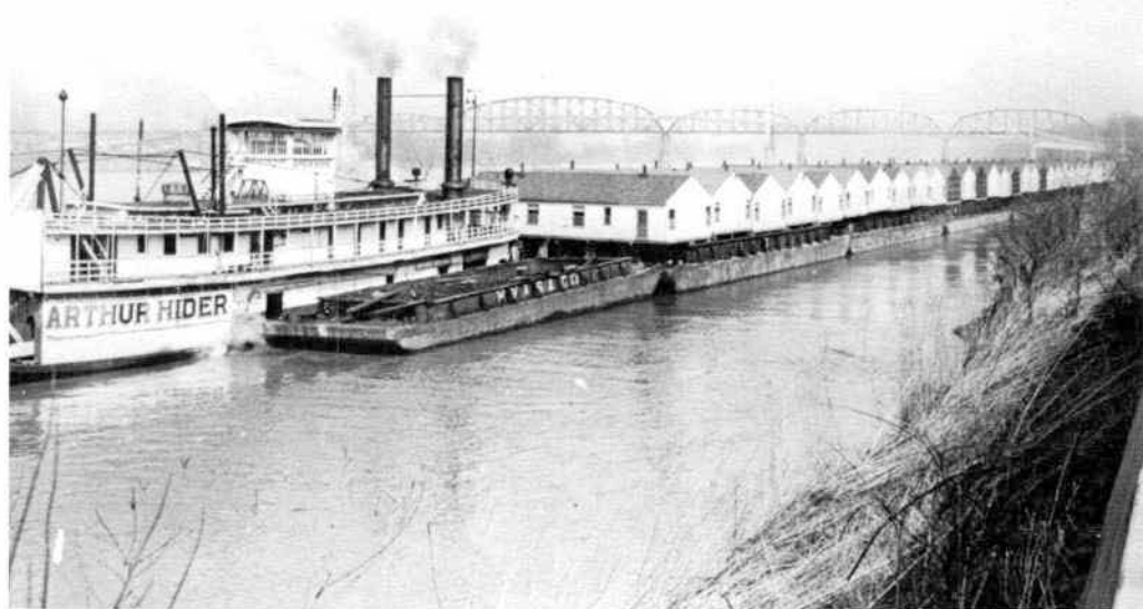
The tow assembled and ready to depart from Point Pleasant. The K&M railroad bridge is in the distance, upriver.
