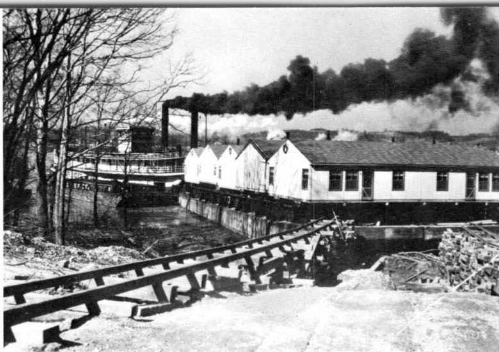
Five double homes loaded and ready to be switched by the HIDER at Point Pleasant.
