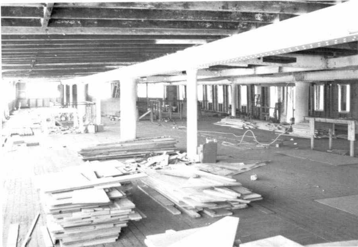
Looking aft from the foot of the interior stairway on the Promenade Deck. This area will be devoted largely to dining area and kitchen. The original diningrooms on the DQ and DK were located on this deck, the meals serviced by dumbwaiter (mechanical elevator) from kitchen and service areas in the hold.
