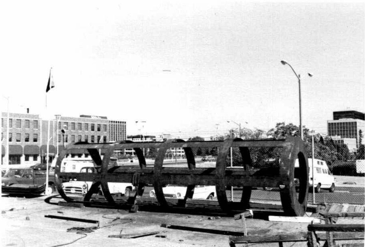
A new smokestack being fabricated at the pier where the KING is presently moored. We have not heard when nor why the original stack was removed.
