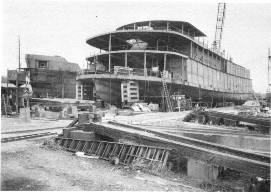
These two photographs taken by Ross Rogers, Jr. show the construction of the GENERAL JACKSON at Jeffboat Inc., Jeffersonville, Ind. in early January. This 245-foot sternwheeler will ply the Cumberland River between Opryland USA and Nashville. The ship at the left in the upper view is a medium-sized ocean-going tanker about ready for launching.
