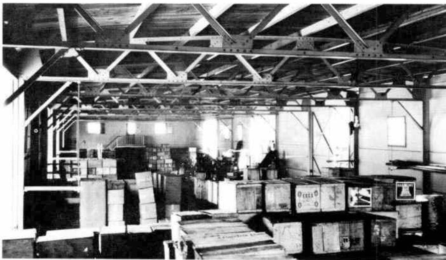
Interior of the Pittsburgh steel wharfboat.
