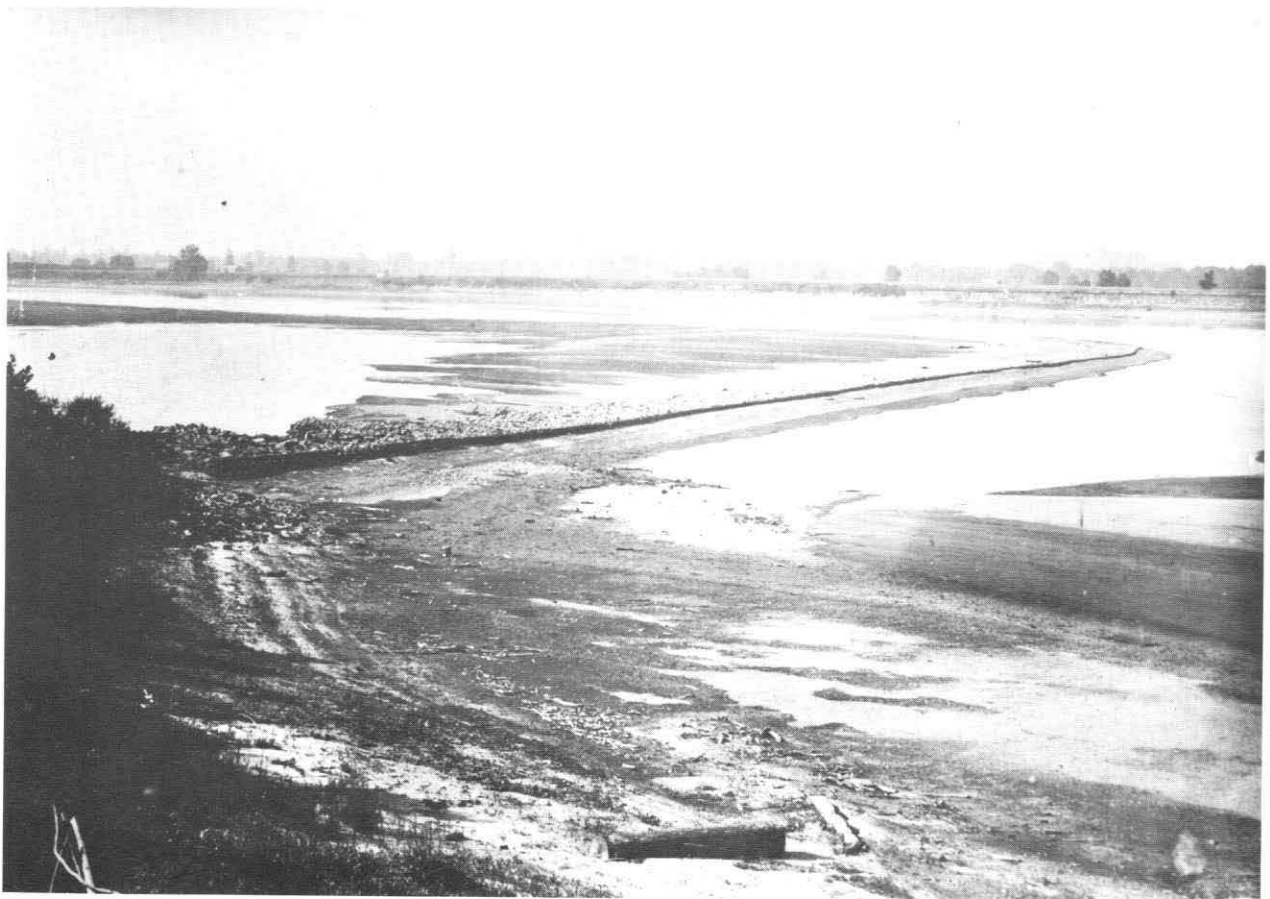
The big towboat EXPORTER greeted the celebrators in newly completed Lock 53, photographed from the CINCINNATI by Capt. Jesse P. Hughes. Slackwater in 1929 outmoded the ingenious system of crib and stone dikes in the Ohio River. One of them below French Islands (below) was 3,500 feet long, photographed during low water from the Kentucky shore on Sept. 8, 1892.
