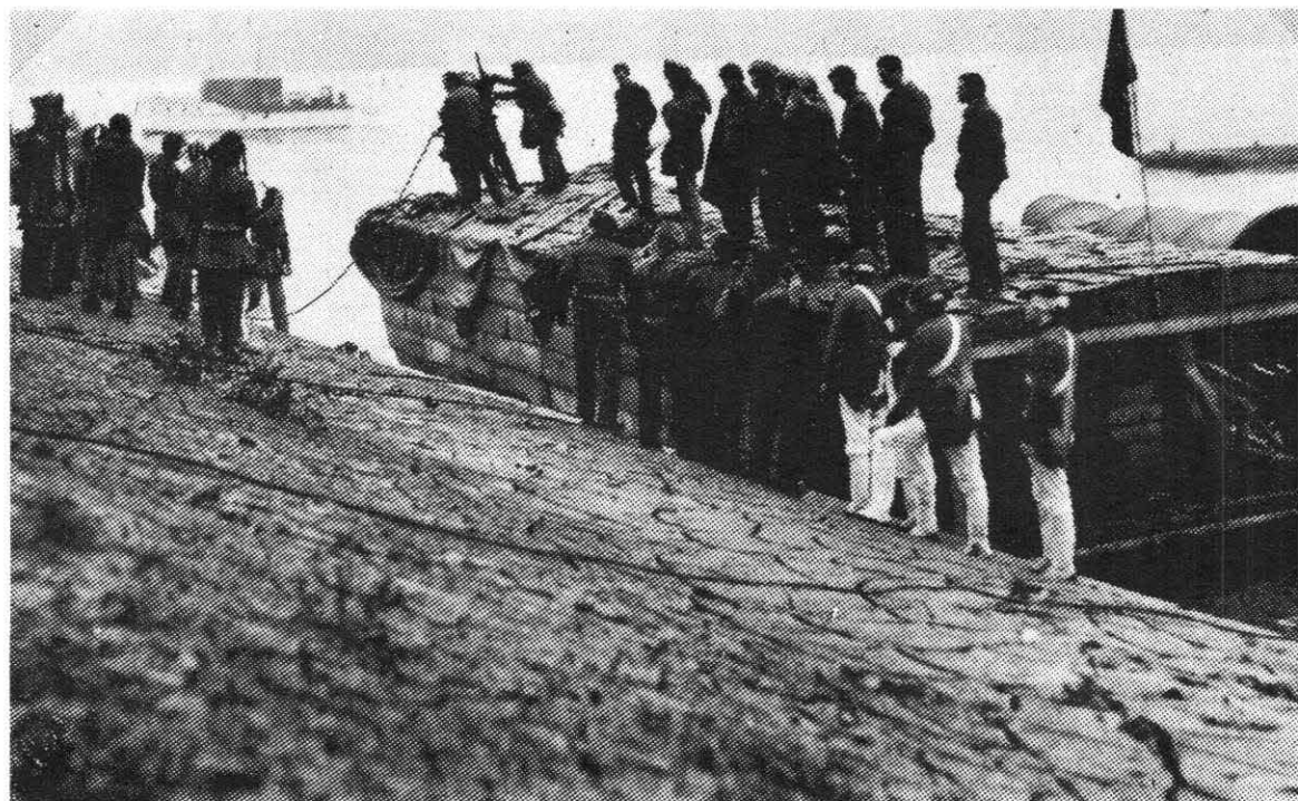
The landing at Marietta on April 7, 1938 at the conclusion of the momentous undertaking originating at Ipswich, Mass. in 1937. This picture is reproduced from a post card made at the time by the late Marietta photographer H. P. Fischer.
