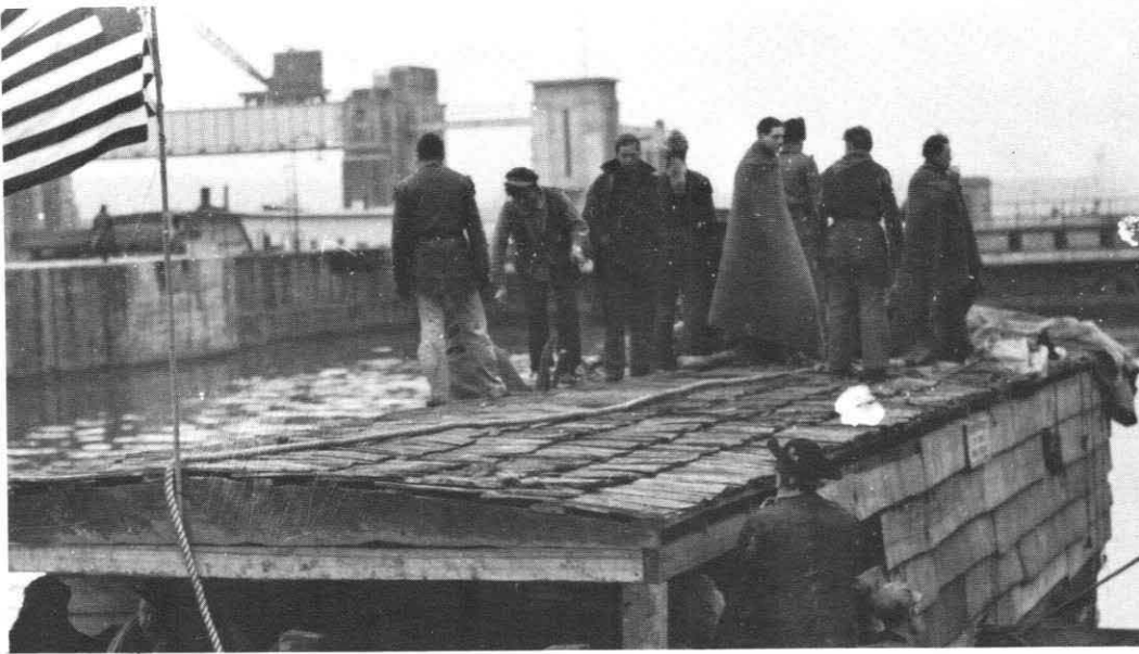
Taken at the Emsworth Locks, Ohio River, in early April, 1938 as the ADVENTURE GALLEY was being locked through in tow of the U. S. Engineer's towboat SHENANGO. The day was windy, rainy and cold.
