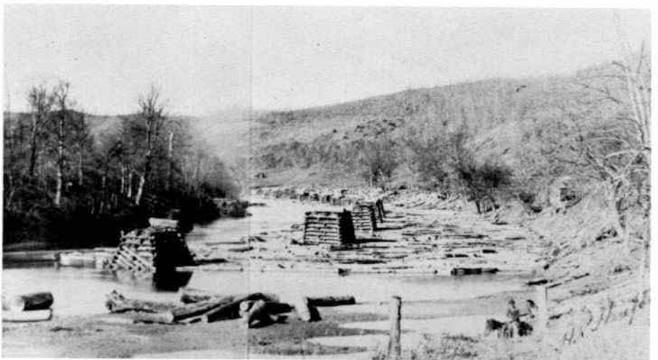
These cribs were above the Lower Falls on Coal River where Lock and Dam No. 2 was located. Today the stone foundations are visible during normal river stages. Herschel Burford, who supplied these prints (see his letter at the left) notes that the original of this view is signed by H. R. Hereford, a St. Albans historian in his time. No explanation is given as to why both pictures were spliced. C. D. Hereford, father of H. R., came to St. Albans on the VICTOR, in August, 1872, and spent the rest of his days there.
