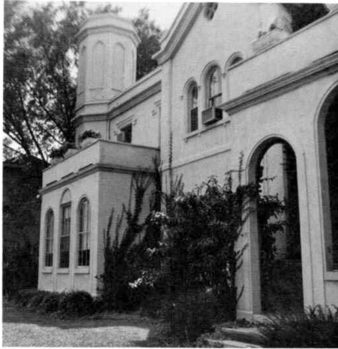
The former David Gibson home entered from Resor Avenue in Cincinnati's Clifton district. Photograph by Lawrence E. Walker taken this past September.
