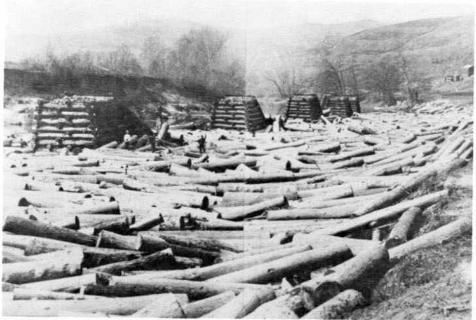
The series of cribs above Indian Creek on Coal River in West Virginia as pictured many years ago. Eventually the wooden upper parts were washed away by ice and flood. The rock foundations remained. When Winfield Dam was built in the Kanawha the new pool barely covered these foundations. Modern pleasure boaters exploring up Coal River, uninformed, often hit them--hard.
