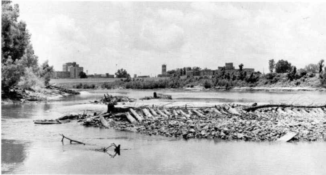
Photo taken in mid September 1972 looking down Red River showing remnants of Bailey's main dam with the gauge showing less than -2 ft. At left is a breach separating the dam remnants from the Pineville shore. The buildings opposite are at Alexandria which "enjoyed" a 22-foot flood about a month after this picture was made.
