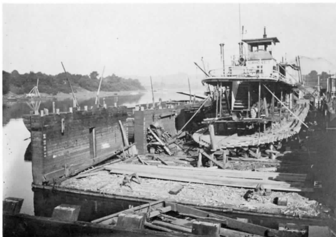
Here is the CRICKET on the docks at Parkersburg, W. Va. when her open hull was decked and a model bow placed. The docks were in the mouth of the Little Kanawha and this is taken looking toward the Ohio. The Parkersburg wharfboat shows across (top center) and above the B&O bridge pier (right) is the ENOS TAYLOR partly visible.
