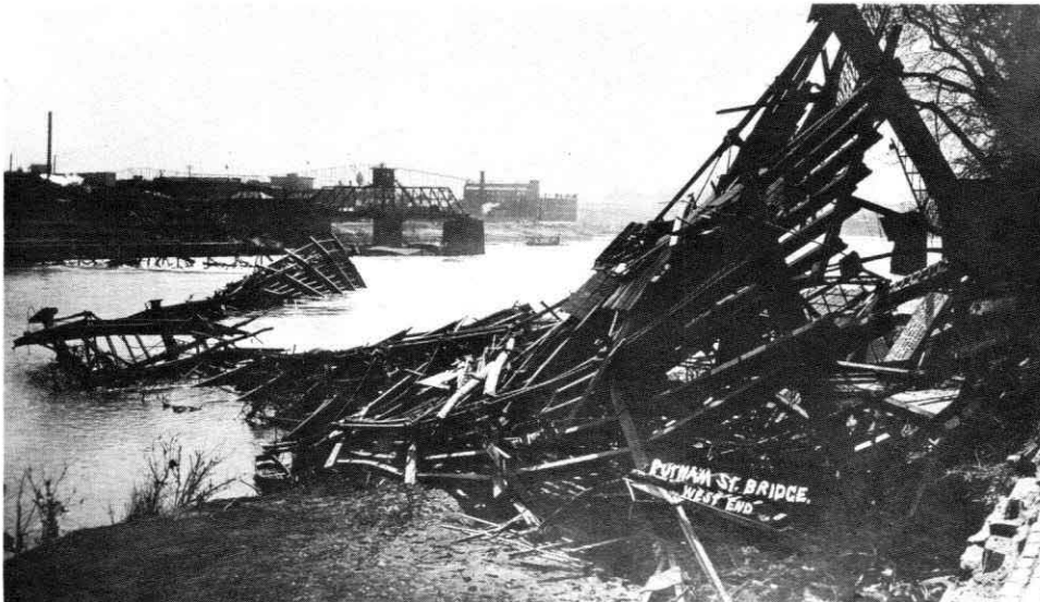
Aftermath of the 1913 Flood in the Muskingum at Marietta. The Putnam Street bridge in the foreground was a mass of ruin. Some of the truss work lodged below Dam No. 1 and was not recovered until the fall of 1968. The swing span of the B&O railroad bridge survived, plainly seen here. Beyond it is the old Nye Foundry, most of which was later torn down, the site now occupied by the U.S. Engineers.
