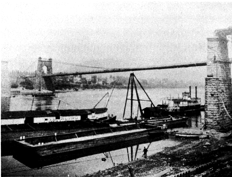
Wheeling, Summer 1891 Story upper right, next column.
