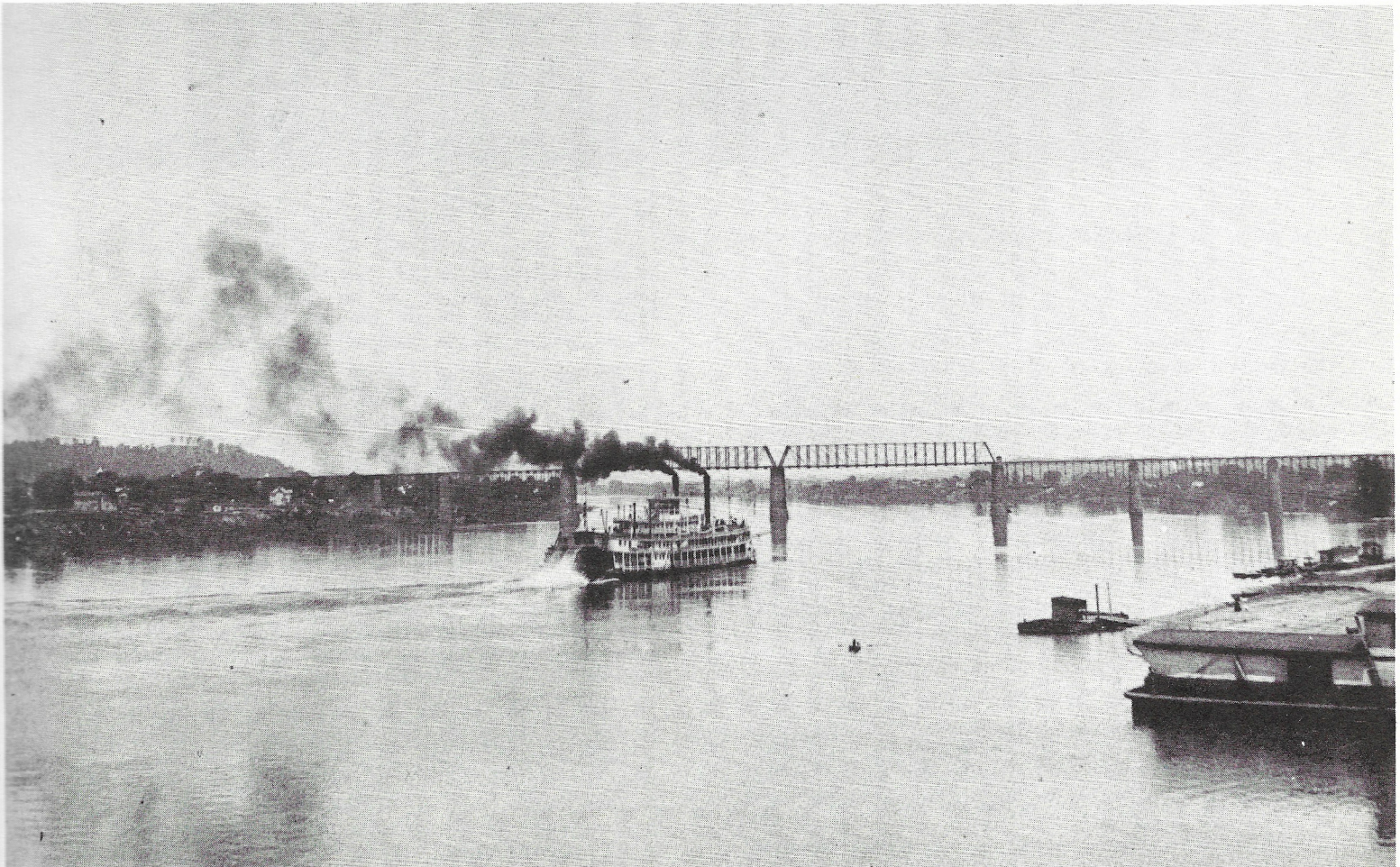
QUEEN CITY upbound at Parkersburg, W. Va. approaching the B&O bridge completed in 1871 with underslung "shore" spans (on right) which later were removed, and replaced with overhead trusses. Wharfboat (extreme right) lies in the mouth of Little Kanawha River, built Murraysville, W. Va. in 1892.
