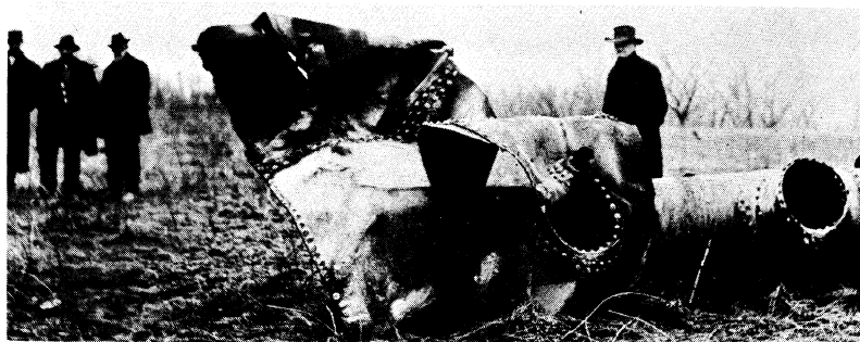
The pilot sailed away to the leeward. This boiler rocketed 450 yards and the concussion broke store windows in downtown Huntington, W. Va. The photo was made at Chesapeake, O. after the towboat SAM BROWN let go on February 2, 1916. Ten killed, four injured.
