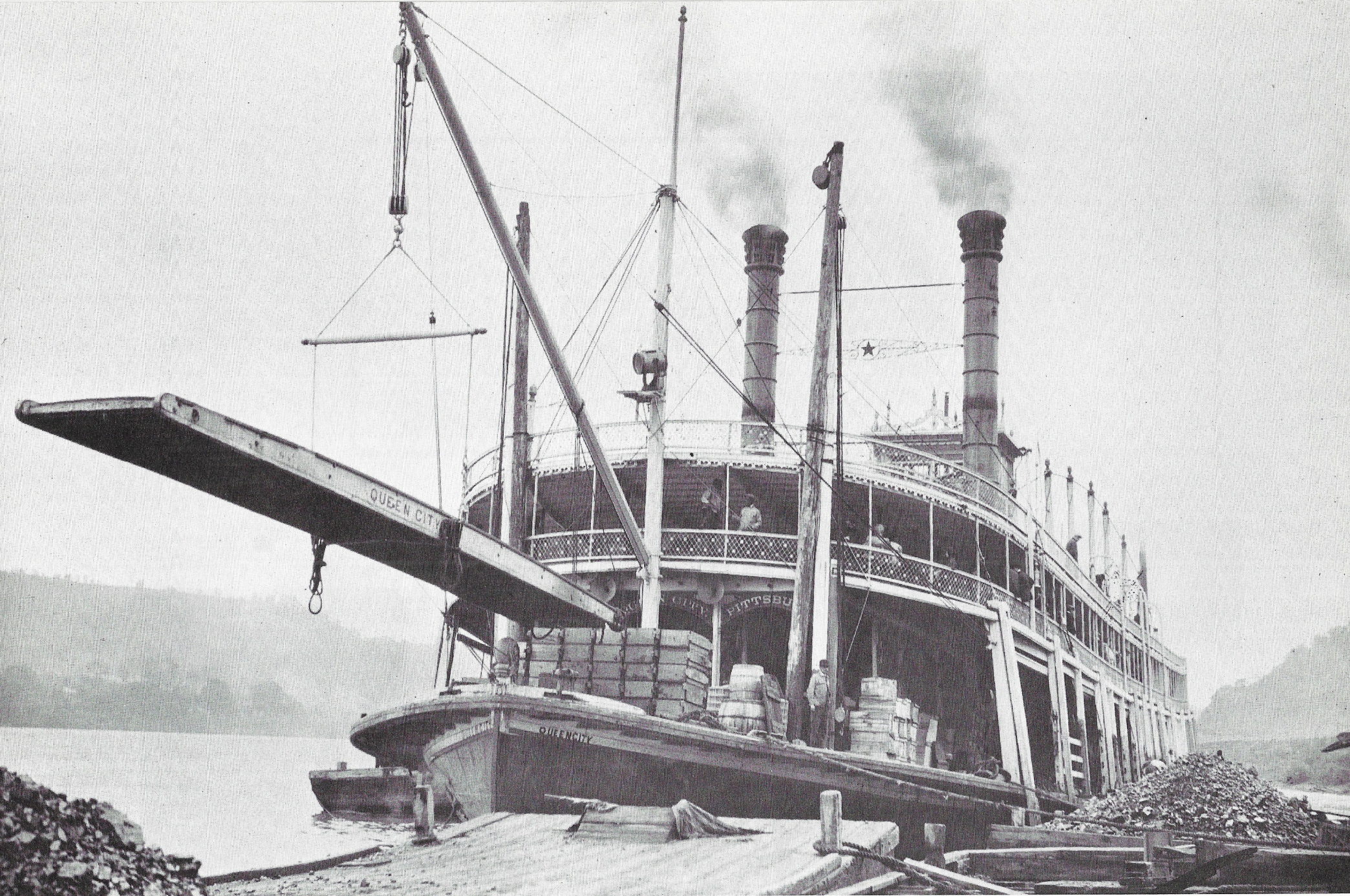
Taking on coal. These Pittsburgh-Cincinnati packets usually fueled at Ashland, Ky., Minersville (above Pomeroy), and Bellaire. We'd judge this is taken at the latter place. The coal was gravity-loaded from a tipple to a deck flat, then hand-shoveled aboard. She is downbound; see the hogshead and a tierce of straw-packed pottery from East Liverpool on the forecastle.
