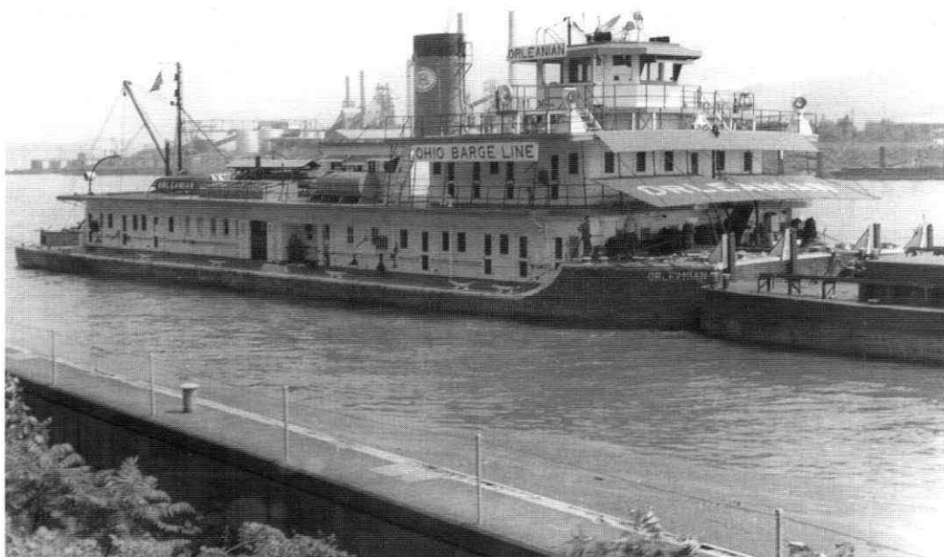
The ORLEANIAN (T1971) was another "DPC" owned by Ohio Barge Line; built as the BATAAN and had been SOHIO LATONIA before renaming in 1949. The high head with abbreviated towing knees, higher than the loaded barge, clearly shows. Photo at Emsworth Lock by W. E. Reed.
